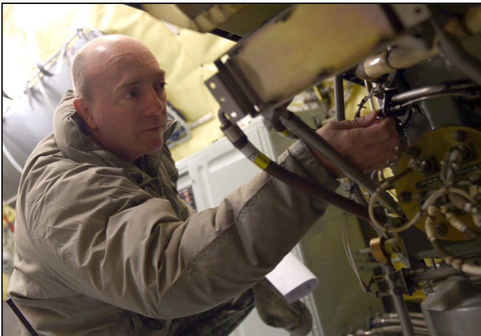
Senior Master Sgt. James Billing, 434th Maintenance Squadron production superintendent, performs a visual inspection on an auxiliary power unit inside a KC-135R Stratotanker at Grissom Dec. 15.
